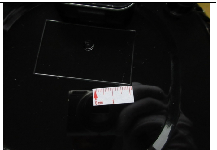
72 Defect-Missing rating label-Critical
